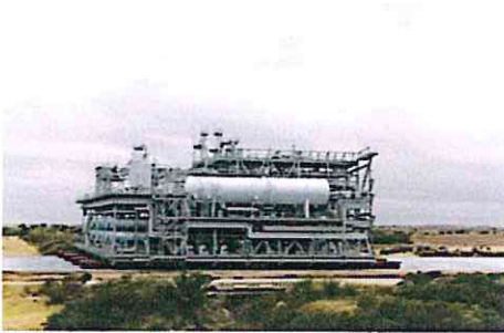
Modules will be transported from the dock to the site via a dedicated heavy haul road to minimize impact on traffic.
