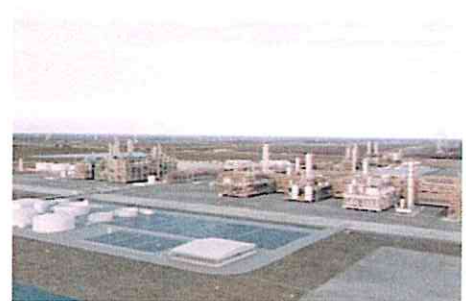
Modularization increases construction efficiency and reduces impact on local infrastructure.
